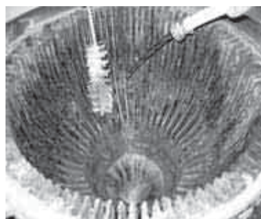
Fig. 9-14 Cleaning the combustion chamber with a water hose
